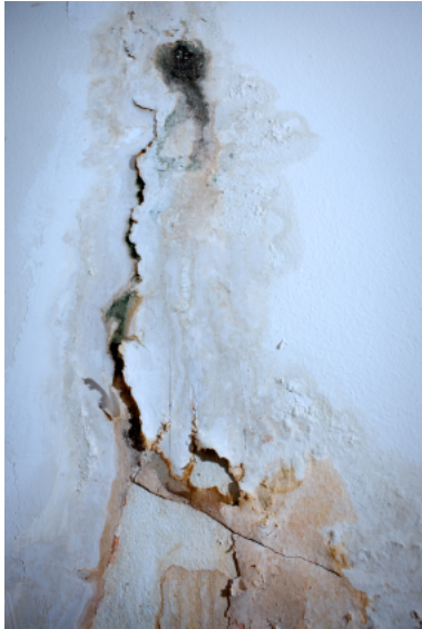
1. Bedroom-Walls-Painted over woodchip paper
