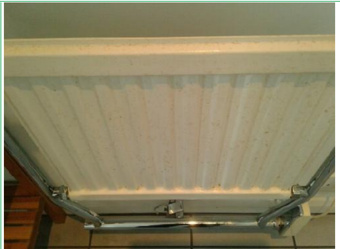
8. Bathroom, 4 bulbs not working, bath sealant mould stained, skirting chipped lhs, sink has no plug, radiator ..
