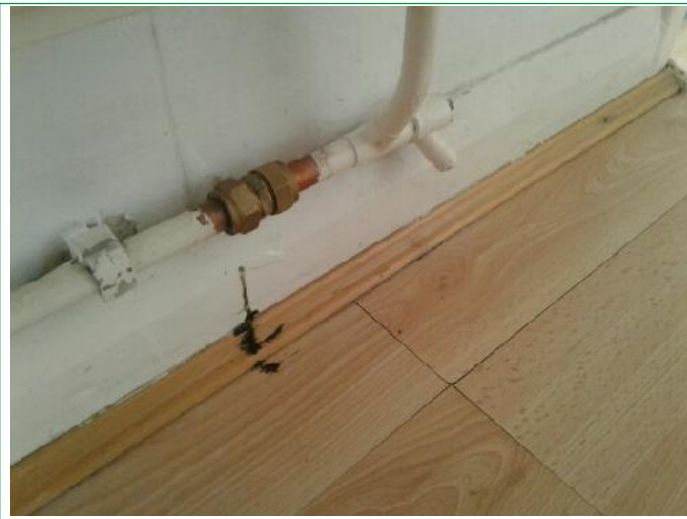
5. Hallway, Walls scuffed mid to lower area LHS, and RHS, entry phone dusty, skirting has black mark under ..
